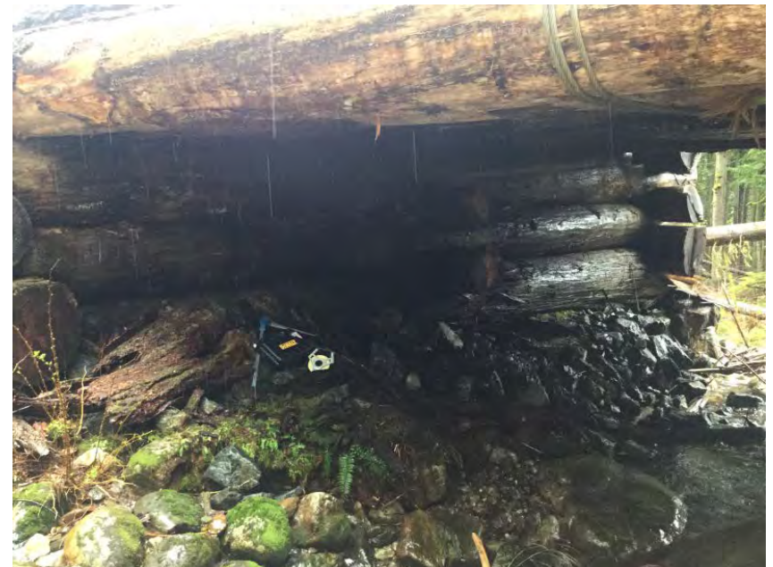
Left Bank Abutment when facing downstream
