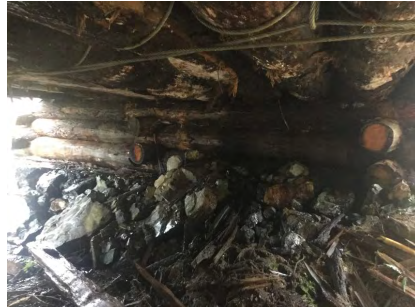
Right Bank Abutment when facing downstream
