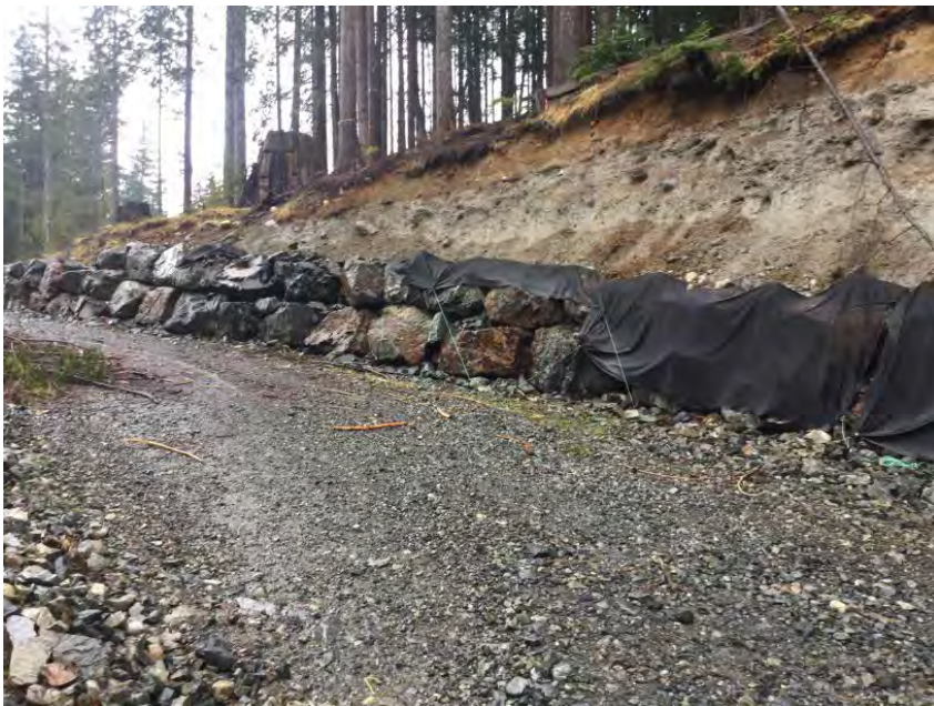
Approach from Right Bank when facing downstream
