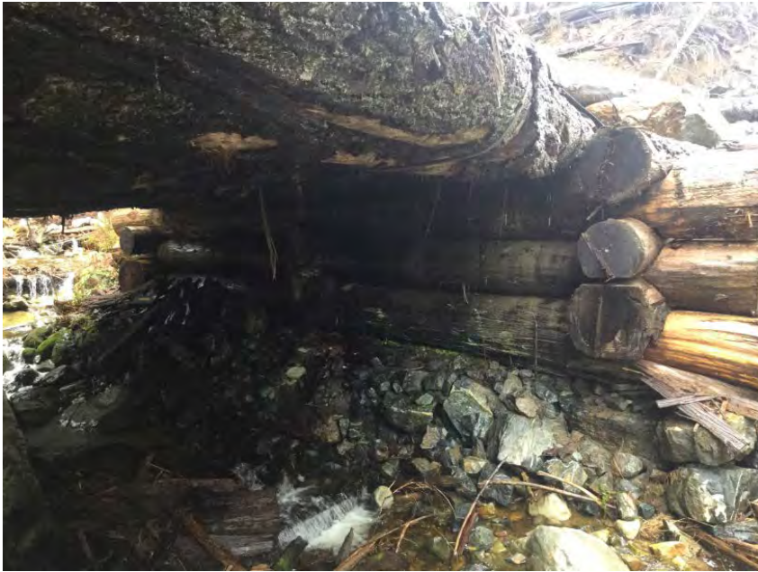
Left Bank Abutment when facing downstream
