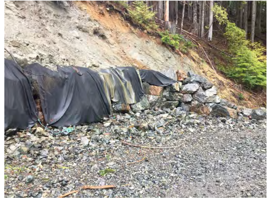
Approach from Right Bank when facing downstream
